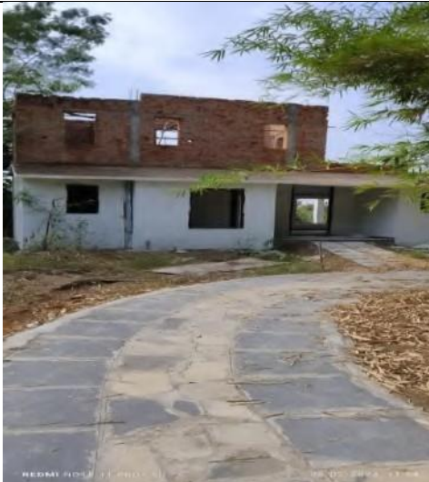
New Construction observed
