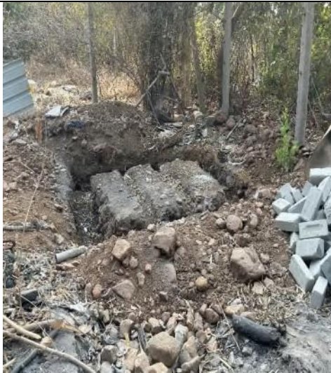
Under construction composting pits
