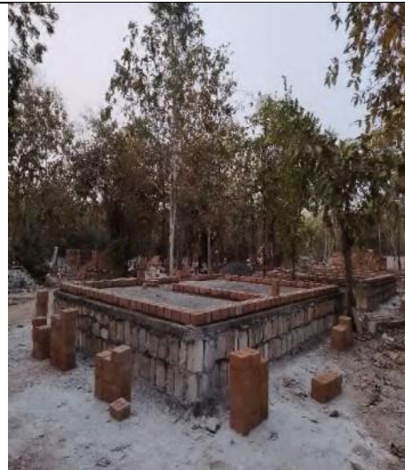
Cottage under construction
