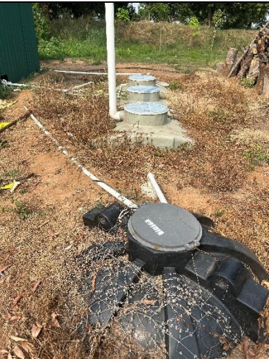
Sewage Treatment Plant
