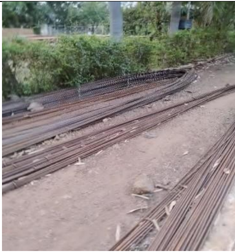
Iron rods used for construction
