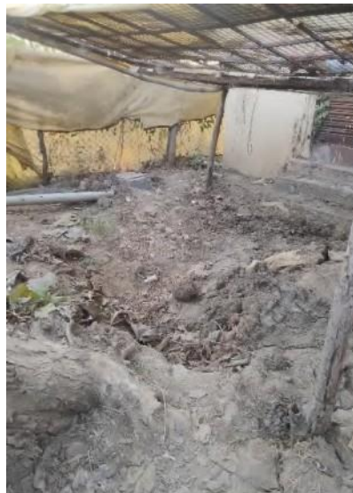
Waste dumping behind laundry room
