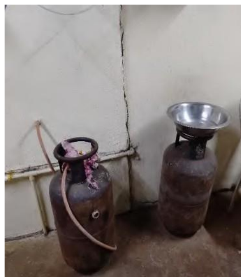
No fire extinguisher near LPG cylinders
