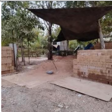
Bricks used for construction
