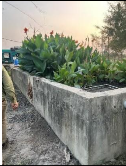
Sewage Treatment Plant
