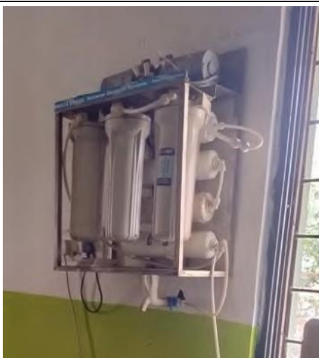
RO filter for water consumption
