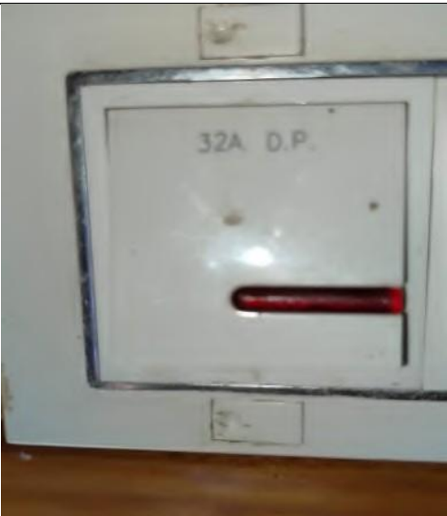
One Button/ Master Switch System
