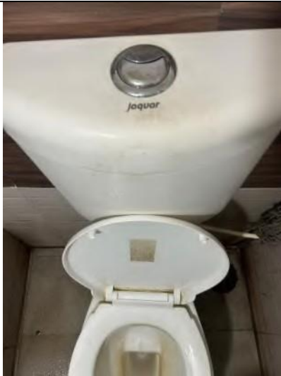
Dual flush system in common washroom
