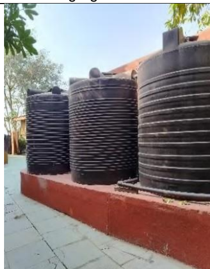
Manual cleaning of septic tanks
