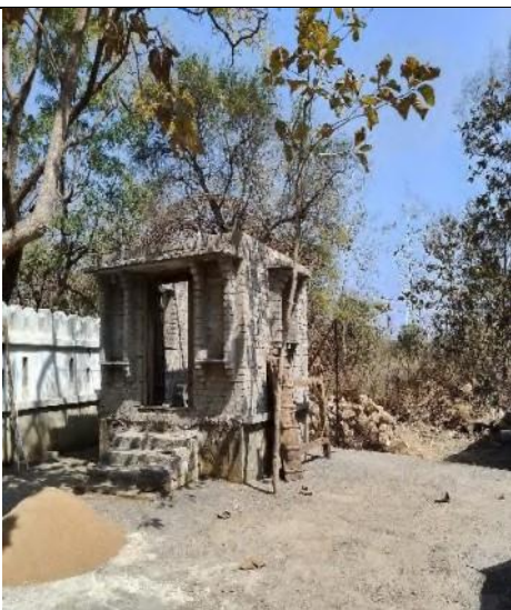
Flyash brick construction
