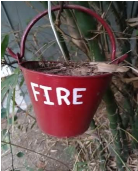
Sand bucket for extinguishing fire
