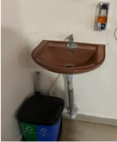
Colour coded bins and soap dispenser
